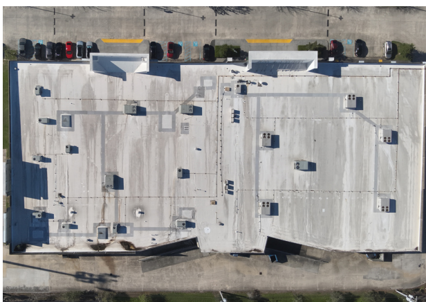
Overall Roof Layout (Nadir 90°)
