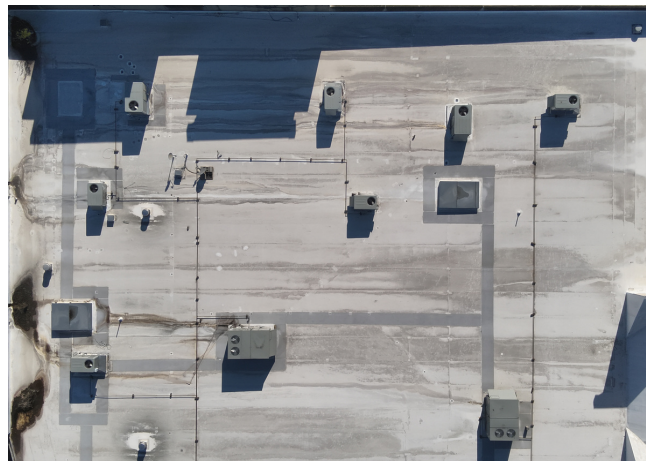
Southeast roof section
