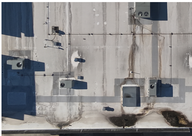
Southwest roof section
