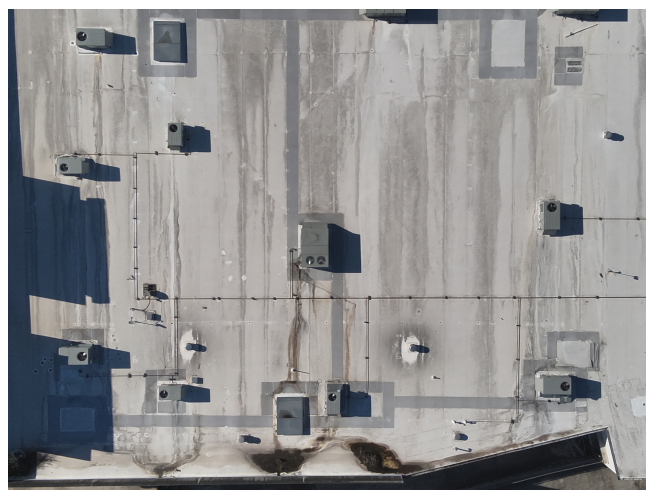
Northeast roof section
