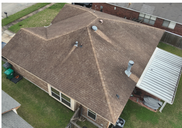
Rear Roof Elevation (Oblique 45°)
