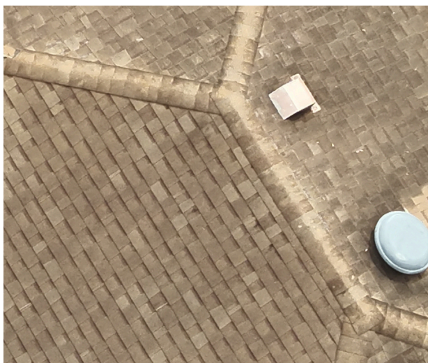
Plumbing Vent & Roof Surface
