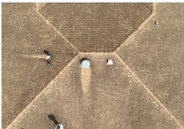
Overall Roof Layout (Nadir 90°)
