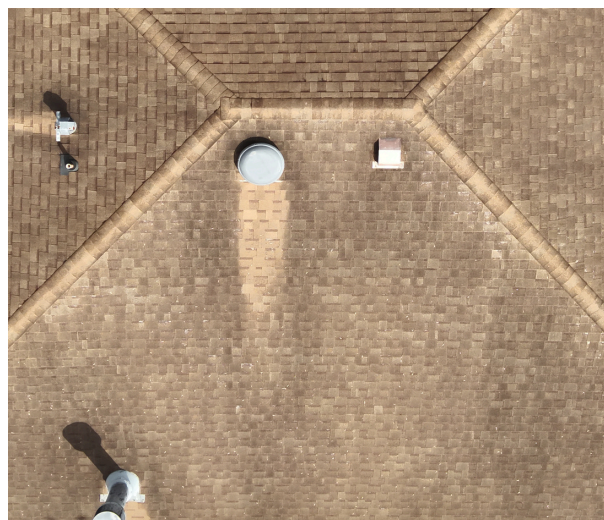
Roof Vent & Ridge Area
