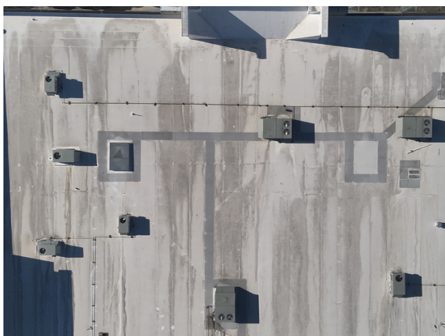
Northwest roof section
