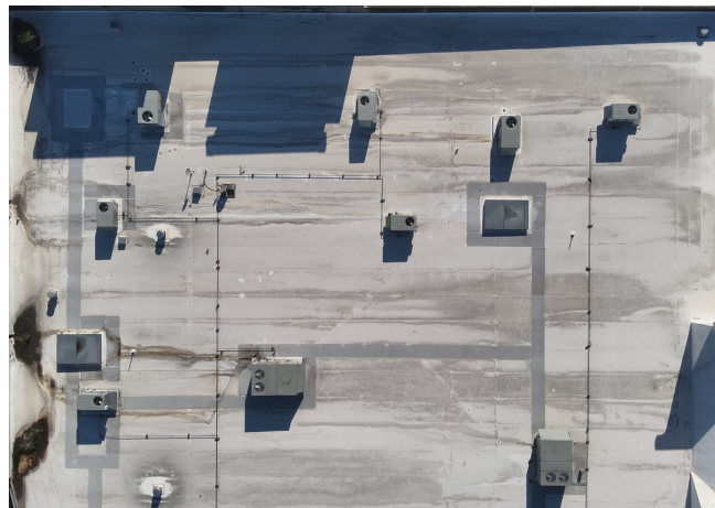
Southeast roof section
