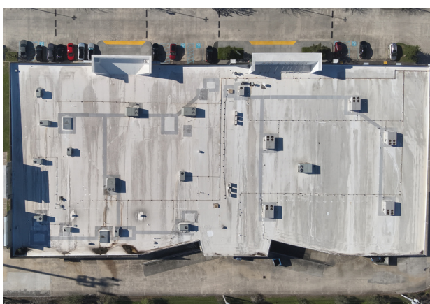
Overall Roof Layout (Nadir 90°)
