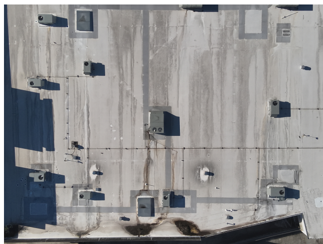
Northeast roof section
