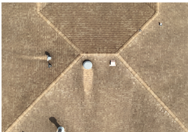
Overall Roof Layout (Nadir 90°)
