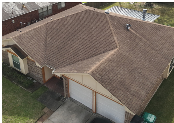
Front Roof Elevation (Oblique 45°)
