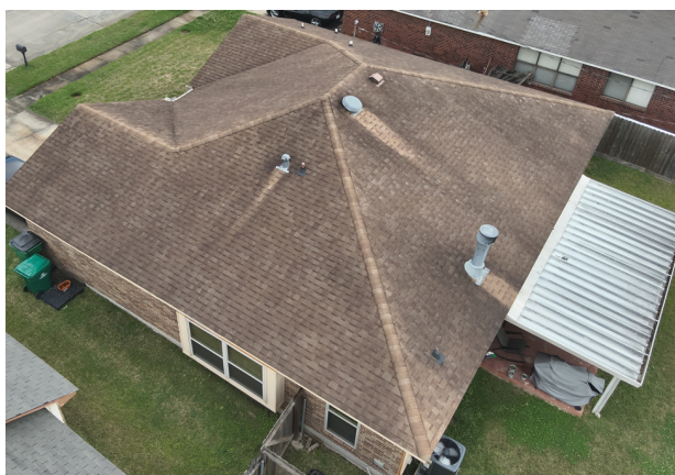
Rear Roof Elevation (Oblique 45°)
