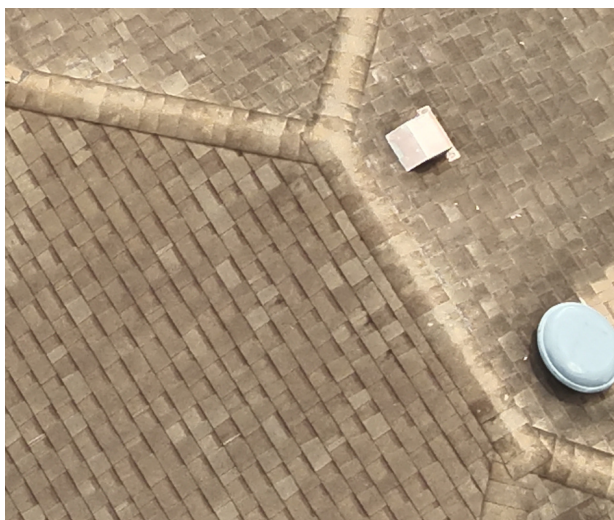
Plumbing Vent & Roof Surface
