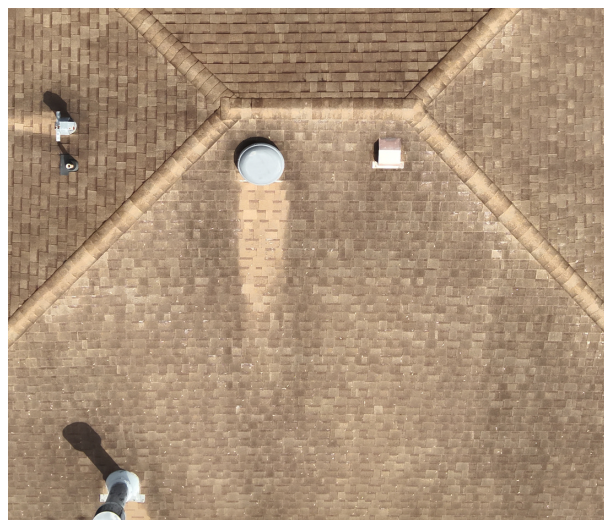
Roof Vent & Ridge Area
